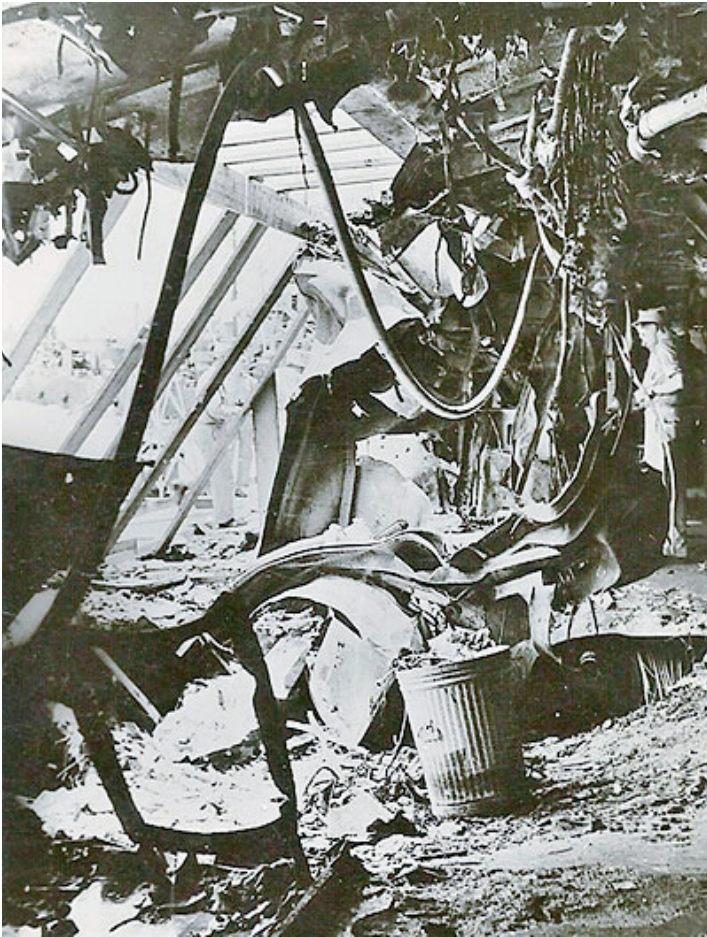
Damage to the USS Comfort . Courtesy of Dorene Lynch.
